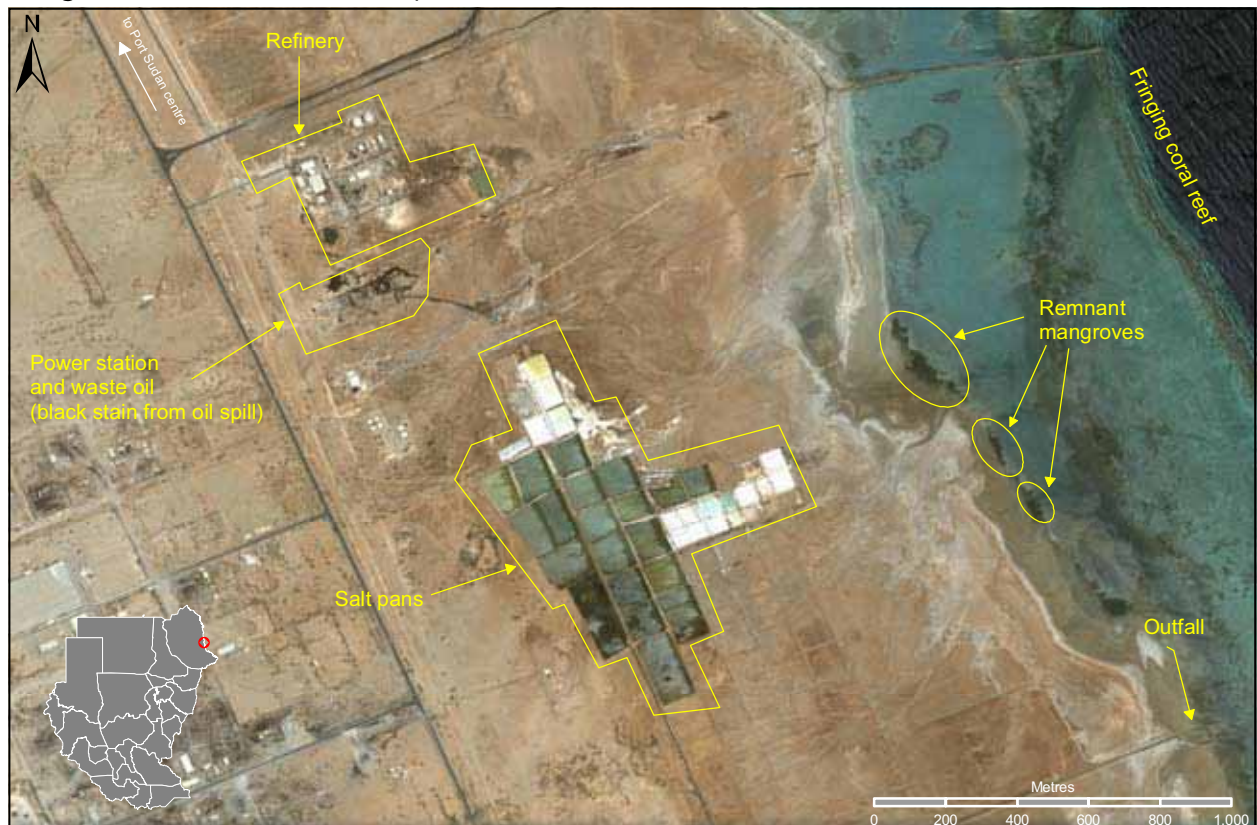
Figure 12.3 Port Sudan power station and salt flats
