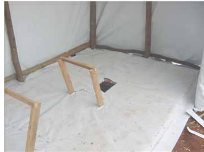
A children's pit latrine built by MSF in a refugee camp in Burundi, 1993.
