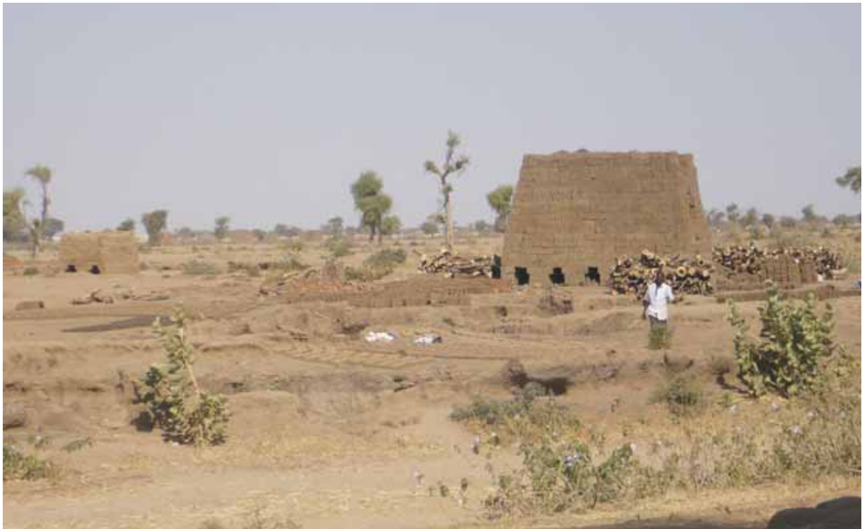
Figure 1. Brickworks like this one in Kass are a major source of demand for firewood
