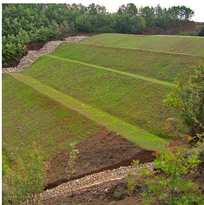
As part of the remediation work undertaken by ENVSEC at the abandoned mining site of Rreshen, Albania, the tailing dam front has been reshaped and a water drainage system has been installed to avoid destabilization of the dam structure
