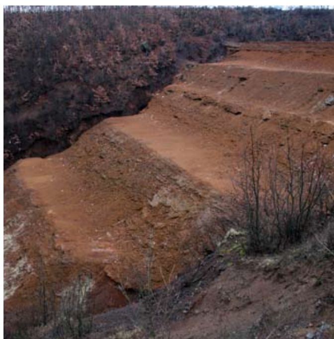
As part of the remediation work undertaken by ENVSEC at the abandoned mining site of Rreshen, Albania, the tailing dam front has been reshaped and a water drainage system has been installed to avoid destabilization of the dam structure
